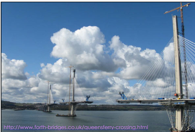
The Queensferry Crossing, Queensferry
