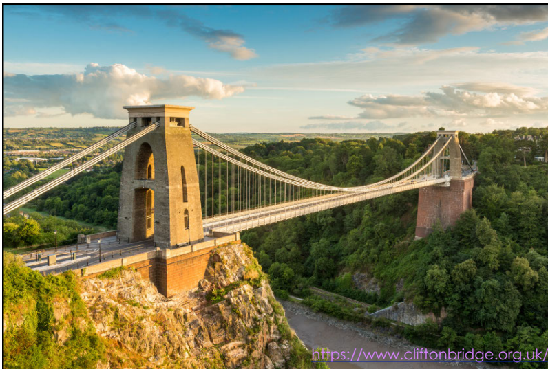
The Clifton Suspension Bridge, Bristol
