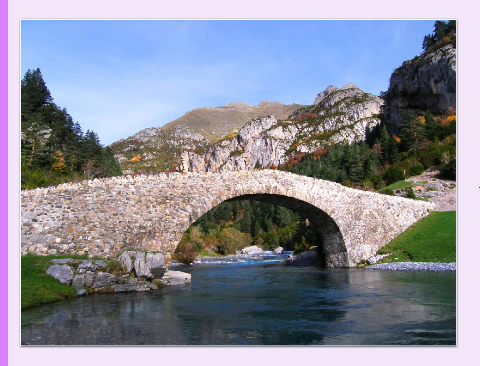
Stones are either cut to shape so they fit neatly together, or fixed in place with mortar. The bridge is built up with more stonework around the arch, usually before the arch frame is removed. This makes the bridge stronger and creates a level surface
