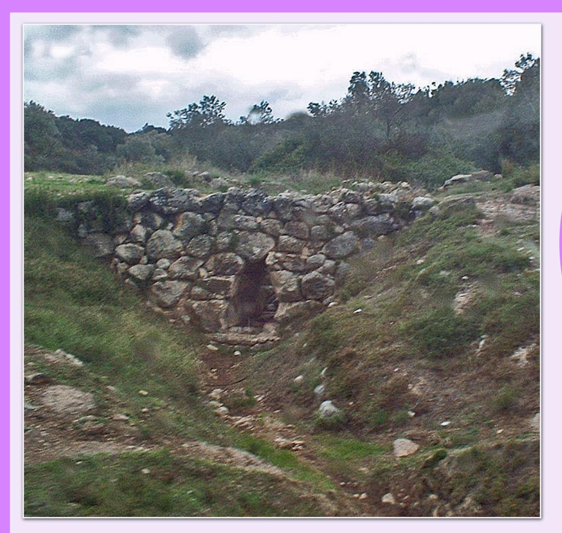
Thin slabs or beams made of stone or brick would break easily, but thick blocks of stone like those used to make this bridge are strong.
