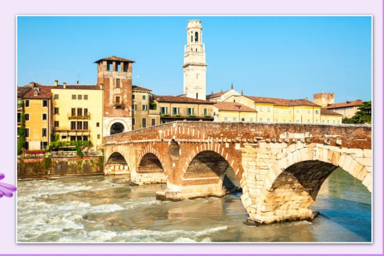
Until developments in technology and engineering meant that engineers could construct large beams made of iron and later, steel or concrete, the best way to construct long, strong and long-lasting bridges was with arches made of brick or stone.
