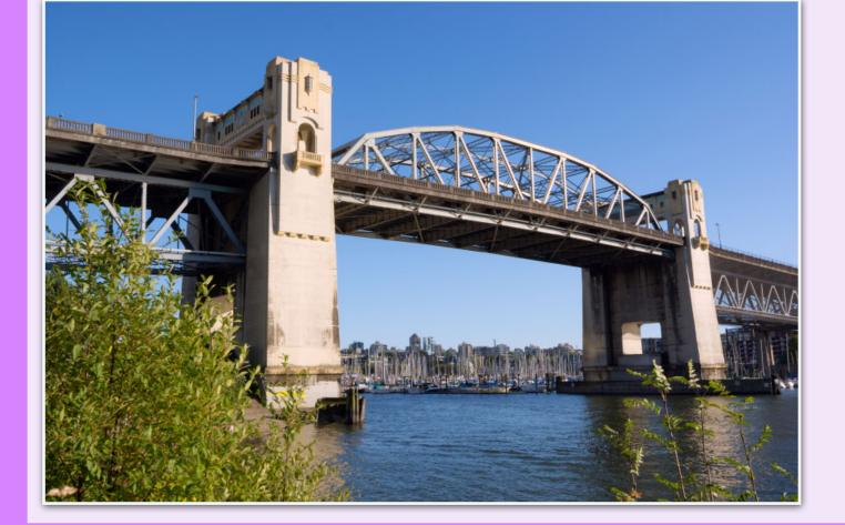
The bridge deck runs through, or on top of the trusses.
