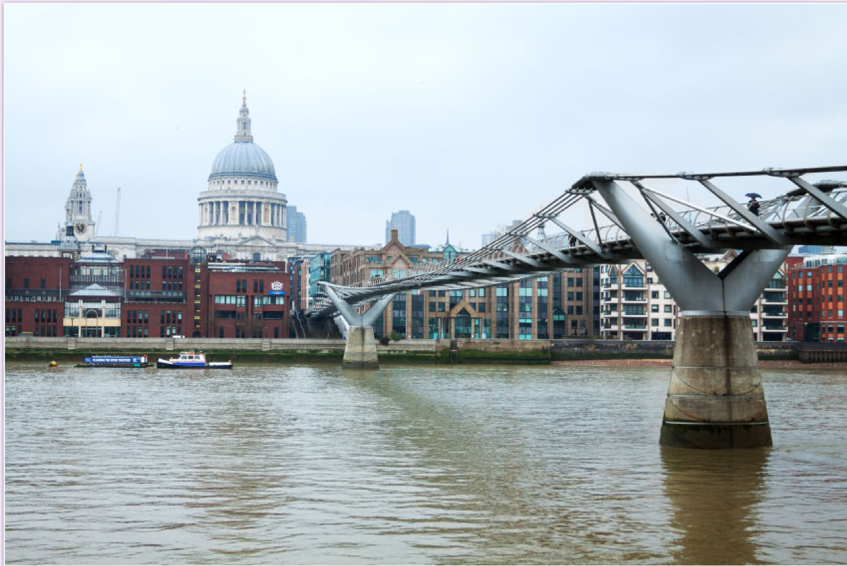
The Millennium Footbridge in London stands on huge, concrete piers.
